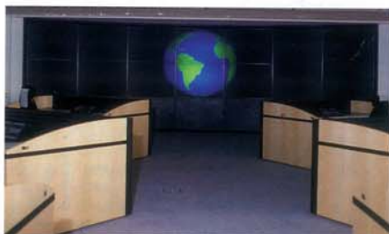
The display at Midlands Electricity's Network Management Centre provides a virtual screen of resolution 8960x2048. Many operators can open windows on the display at the same time. The photograph was taken prior to the Centre becoming operational.
